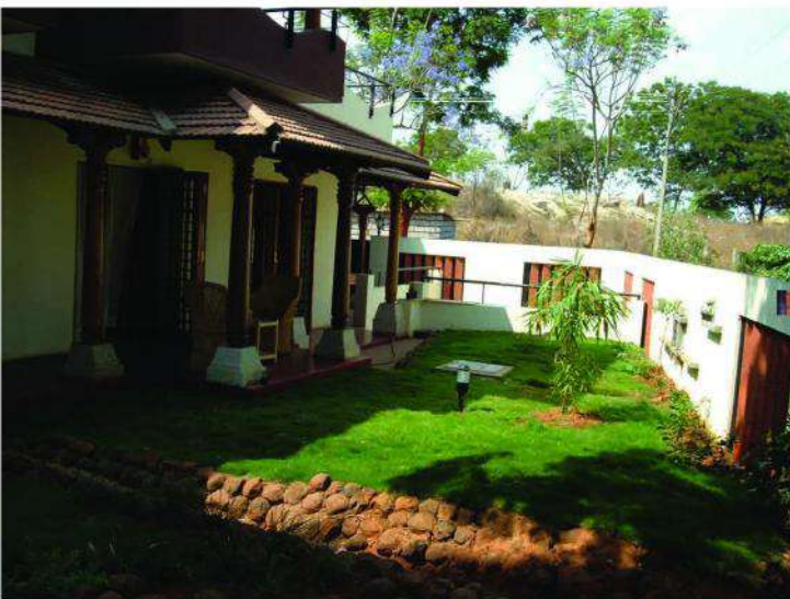
Trayee - Holy trinity is a blend of an old courtyard house with the economy of duplex apartment. Wooden pillars with stone bases were brought from handalagera. The liberal use of skylights in trayee enlightens the whole space.
